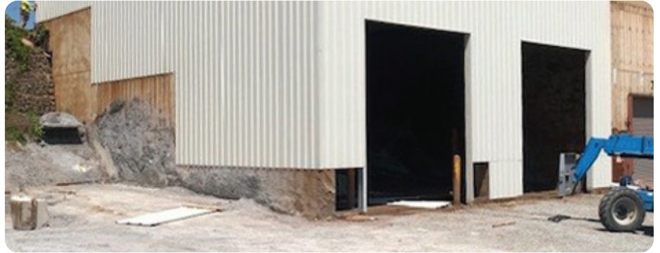
Yukon's containment building receives new application of siding on two bays
