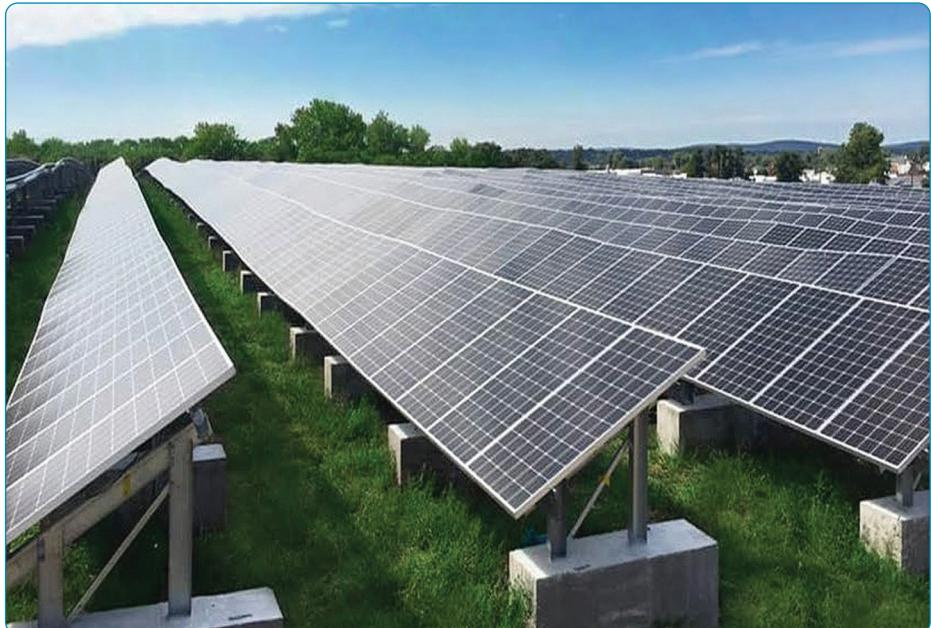
*Ballasts are used to support solar panels that are placed on landfills. This construction method avoids digging, and thus prevents damage to cap systems*
