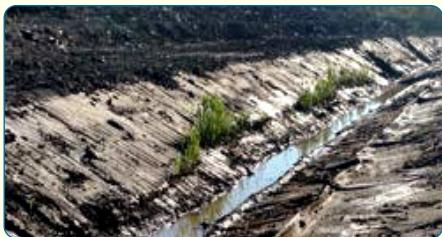
The newly constructed perimeter trench will minimize rainfall recharge into the landfill and facilitate leachate collection.
