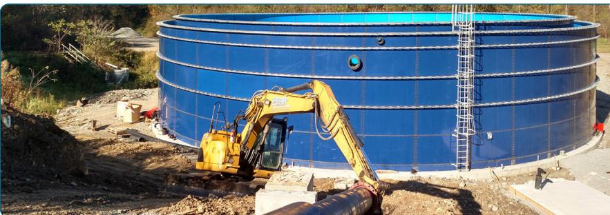
A new storage tank will hold more than one million gallons of leachate from Landfill 6. The leachate drains from a collection system underneath the waste. It is processed in an on-site wastewater treatment facility.
