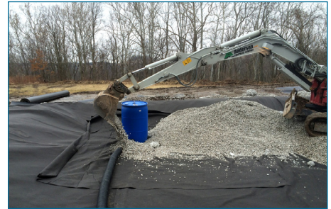
Above, operators at MAX prepare a staging location for used plastic liners from drilling sites. The staging location itself is required to be lined so that accumulated storm water can be collected and sent to the facility's permitted wastewater treatment plant. Liners stored at the site are destined for recycling.
